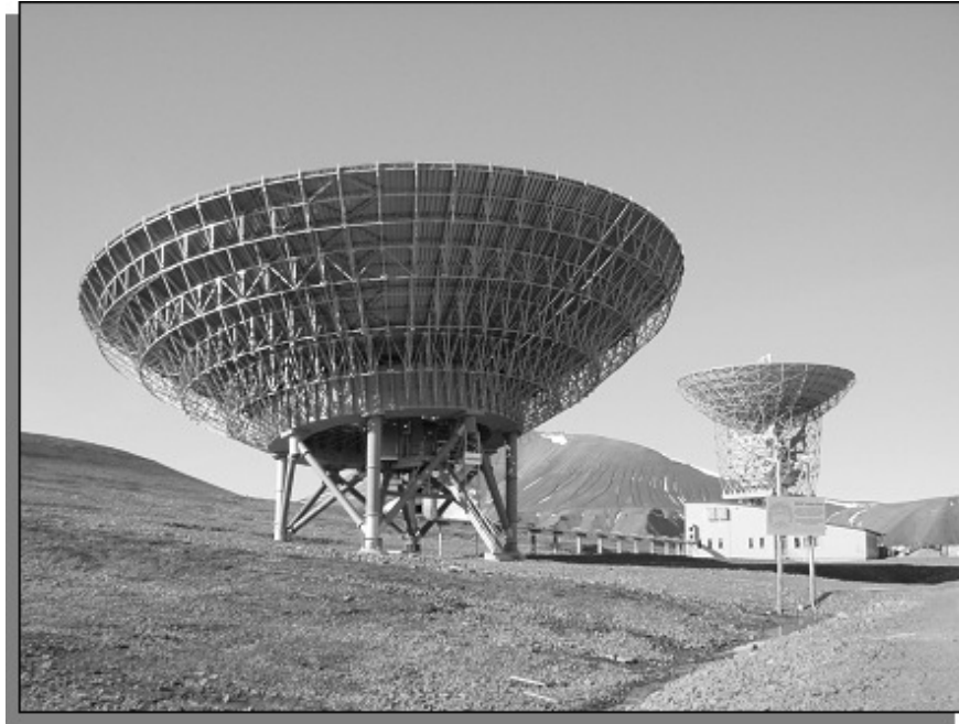
Figure 12.14.: The 42m and 32m 500 MHz EISCAT Svalbard Radar parabolic antennas. The one in the background is fully steerable, while the closer one points along the geomagnetic field line about 8.5 degrees from the zenith. Credits: EISCAT
